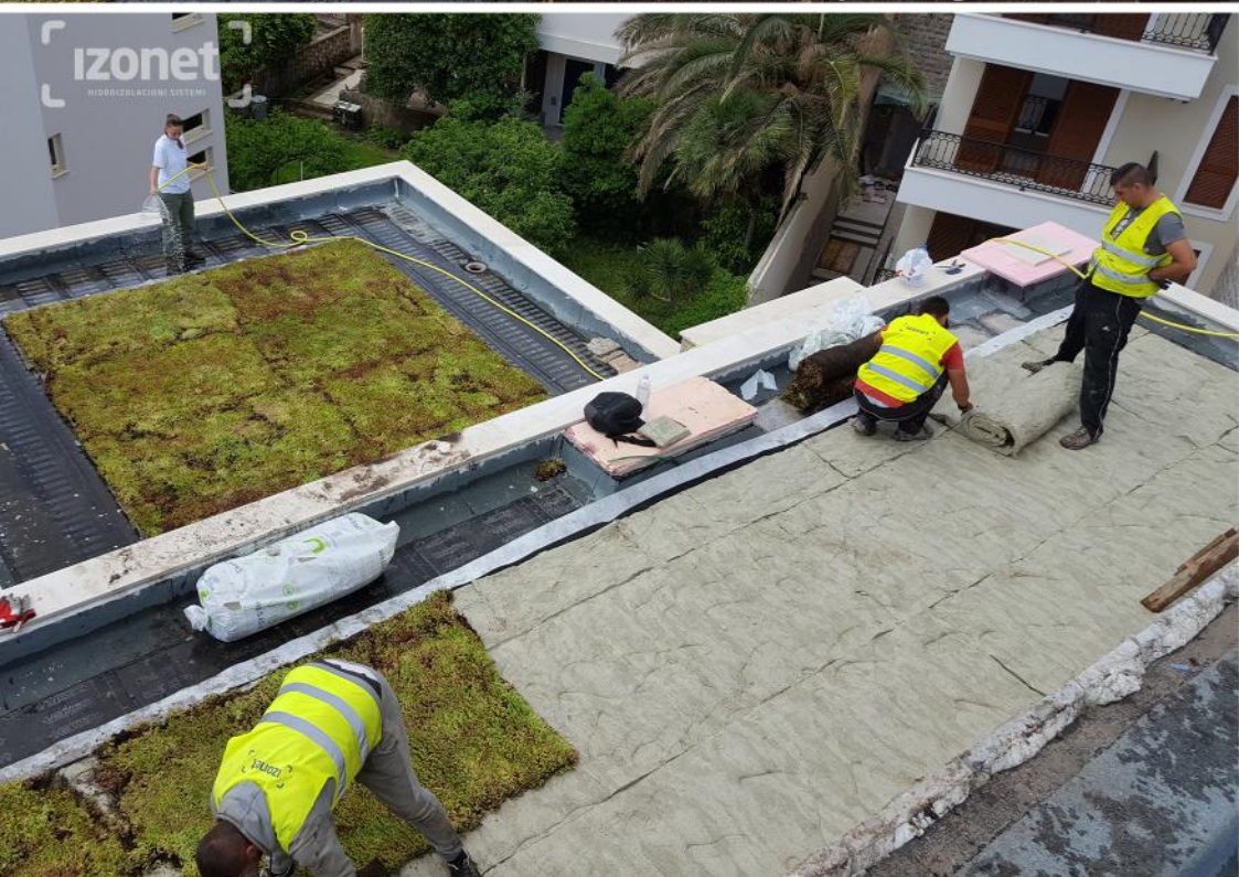
Photos from our construction site where we successfully made green roof.
